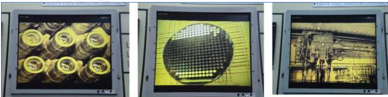
Camera Images Displayed in Control Room
